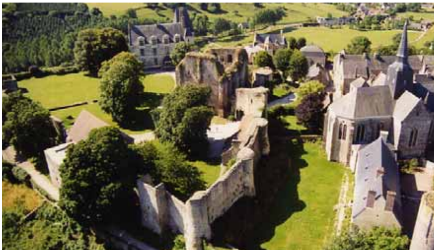
Aerial view of the fortress of Sainte-Suzanne.
