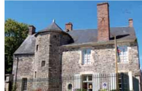
The Butte Verte manor. It was built at the end of the Middle Ages but the windows of the first floor were modified in the 18 th century. The manor shelters nowadays the Tourism Office.
